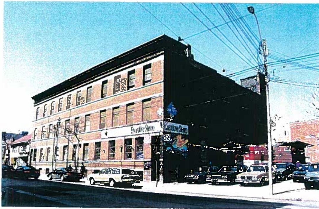
Exterior View Prior to Renovation
